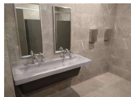
Our new restroom facility at the town park
